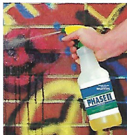
Spray tagged surface with Phase II Cleaner.
